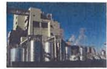
INDUSTRIAL AND WASTE TREATMENT
